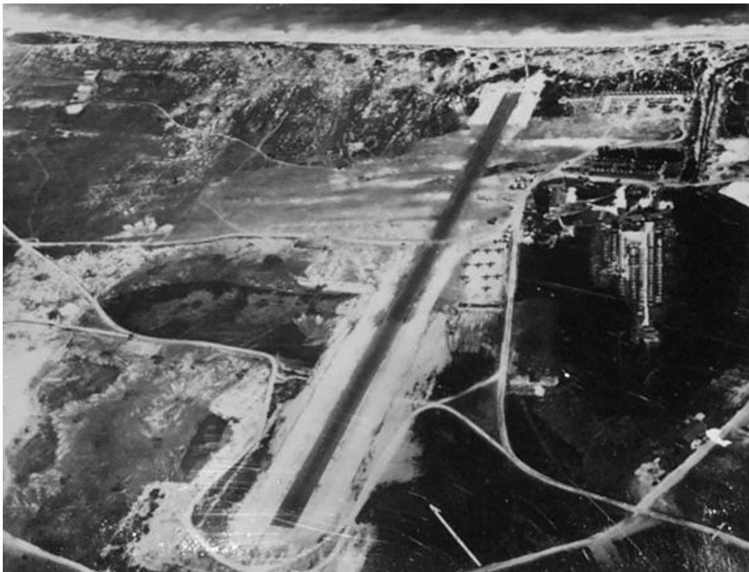
Aerial view of Bellows Field, 27 October 1941, P-40, O-47 and P-26 aircraft are visible, USAF photo
