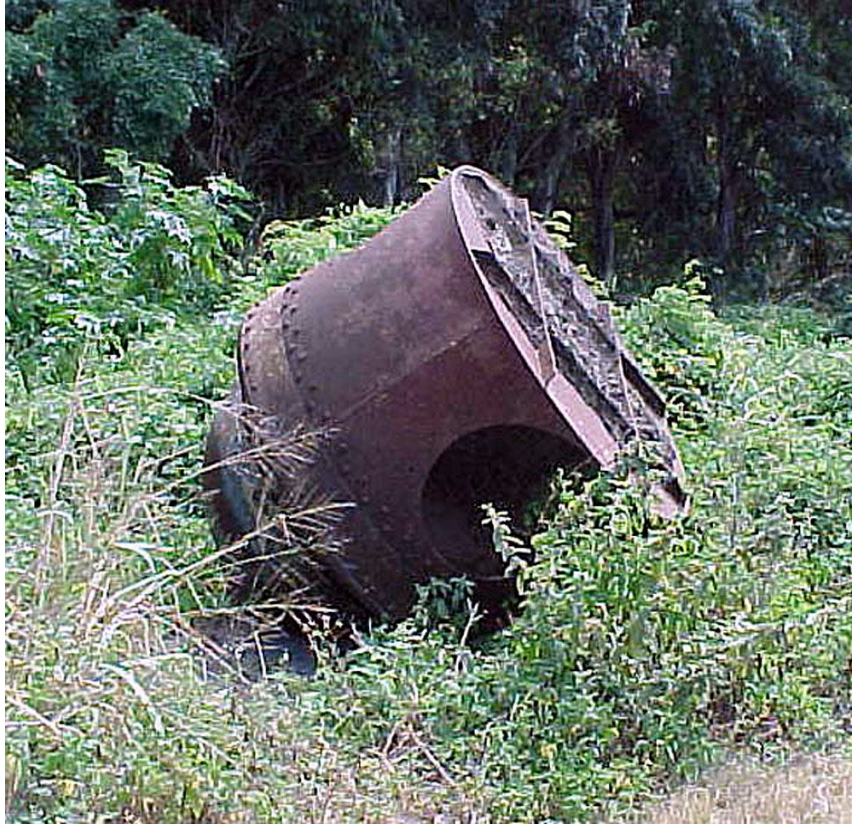
Metal turreted pillbox (Feature G) at Dillingham M.R. Author
