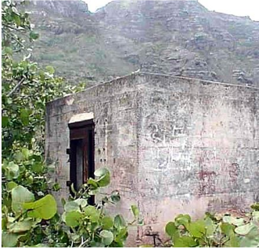
Photo depicts the doorway at the east side of Feature 1A. Author
