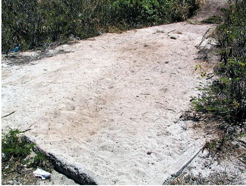
Concrete foundation (not categorized) several yards southeast of Feature 1A. Author
